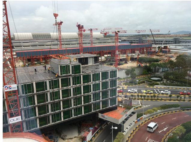
Photo credit: Singapore Building and Construction Authority
