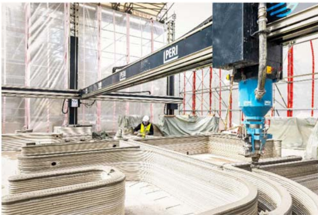
FIGURE 8.44 BOD2 3D printer in operation. Credit: PERI.
