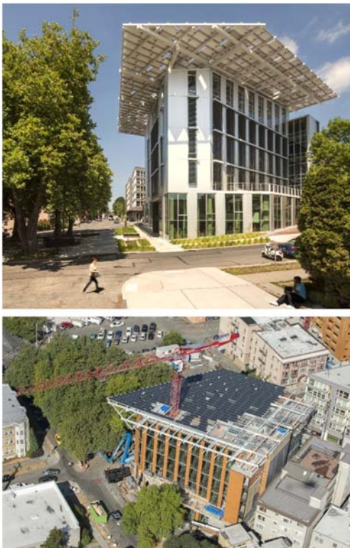
FIGURE 12.7 Bullitt Center, Seattle. Courtesy of Miller Hull Partnership.
