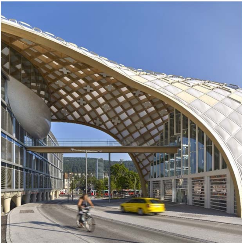
FIGURE 6.51 Swatch HQ, Biel. Courtesy of Shigeru Ban Architects, photo by Didier Boy De La Tour.
