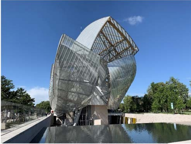
FIGURE 6.27 Louis Vuitton Foundation by F.O. Gehry (photo by the author).
