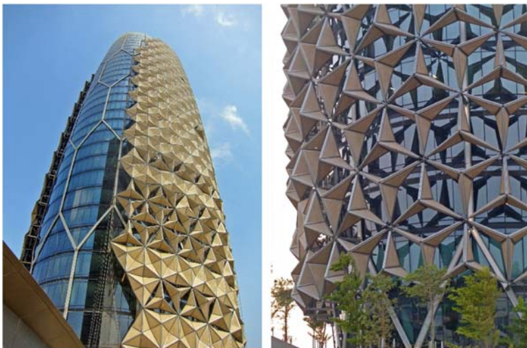
FIGURE 10.3 Adaptive façade of Al Bahar Towers, Abu Dhabi. Courtesy of Arup.
