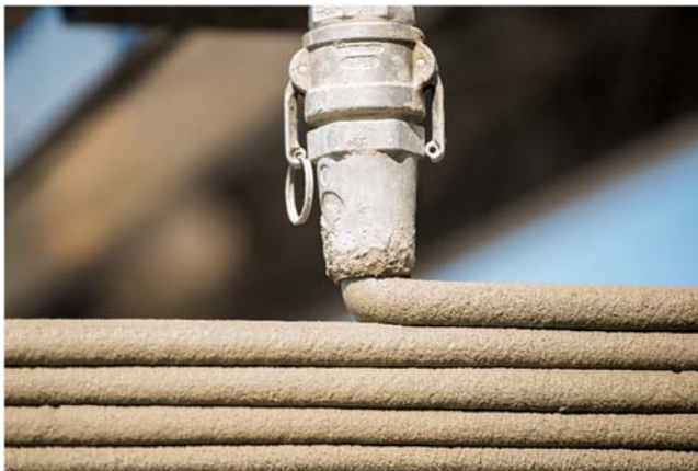
FIGURE 7.9 3D printed concrete nozzle. Courtesy of ICON, photo by Regan Morton Photography.
