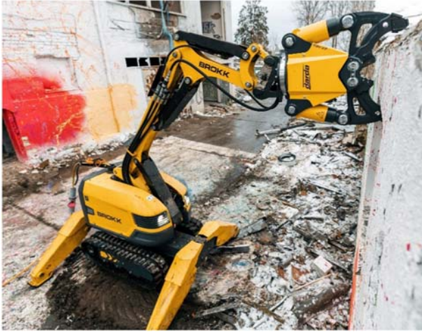
FIGURE 8.4 Brokk teleoperated demolition robot. Courtesy of Brokk.
