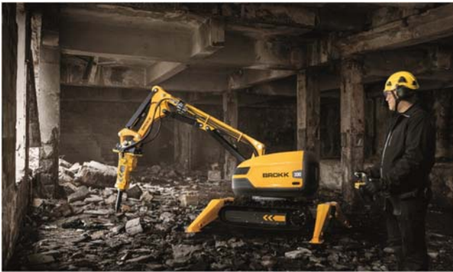
FIGURE 3.11 Single task demolition robot. Courtesy of Brokk.
