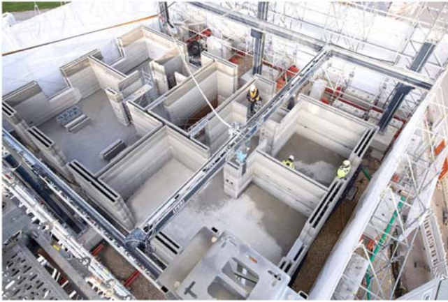
FIGURE 8.45 3D-printed house in Bavaria. Credit: PERI.
