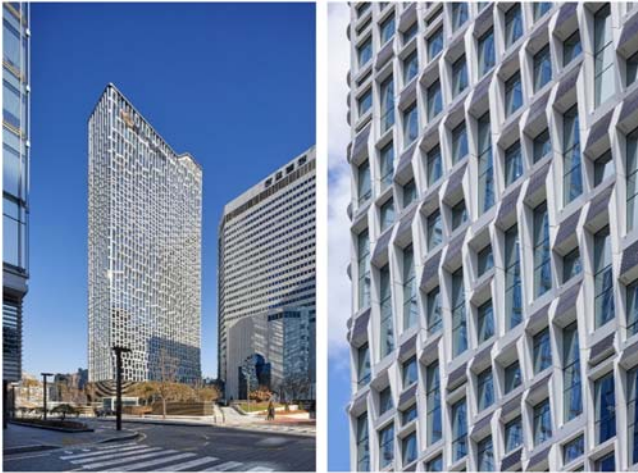
FIGURE 12.11 Hanwha HQ Building. Courtesy of UNStudio, ©Rohspace.
