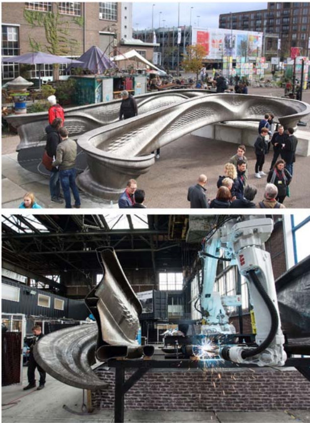
FIGURE 8.31 3D-printed steel bridge. Courtesy of MX3D, photos by Adriaan de Groot (top) and Oliver de Grujter (bottom).
