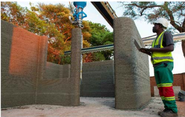
FIGURE 8.46 3D-printed house in Malawi with BOD. Credit: 14trees.
