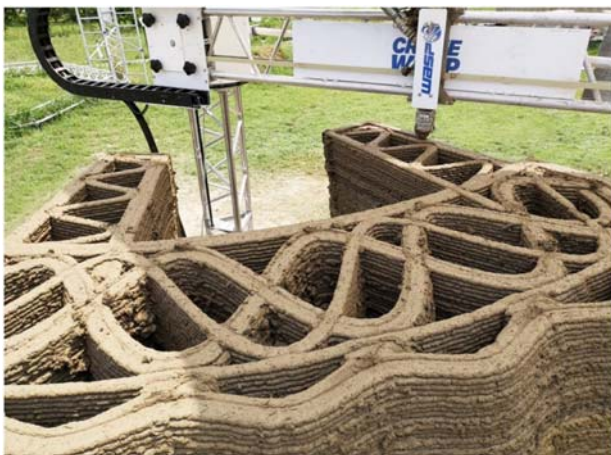
FIGURE 8.33 3D-printed cellular structure. Courtesy of WASP.
