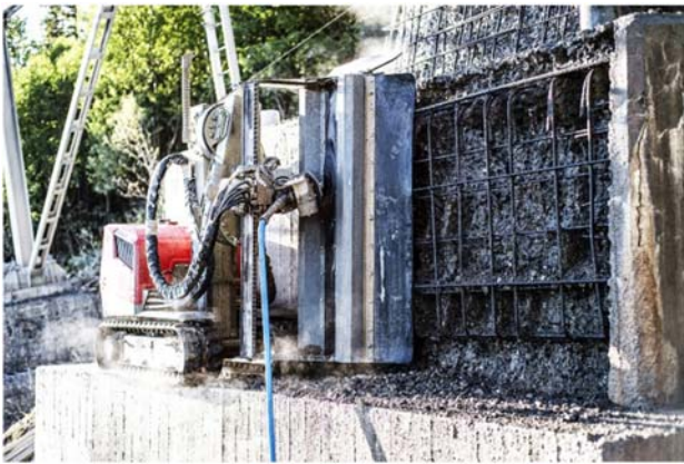
FIGURE 8.5 Hydrodemolition robot. Credit: Aquajet Systems.
