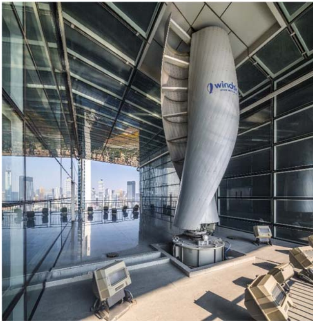
FIGURE 12.24 Savonius VAWT inside Pearl River Tower. Courtesy of SOM.
