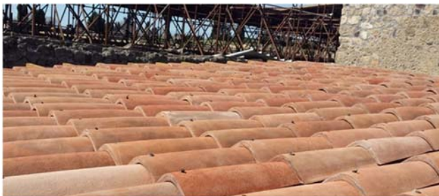
FIGURE 7.39 Mimetic PV roof tiles in Pompeii Archeological Park. Courtesy of Dyaqua.
