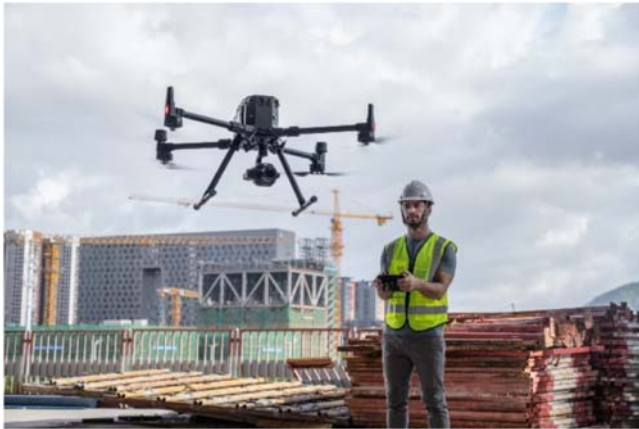
FIGURE 3.8 Construction site monitoring with drones. Courtesy of DJI.
