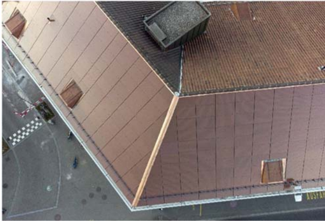
FIGURE 7.38 Mimetic PV roof on an historical center. Courtesy of Solaxess.
