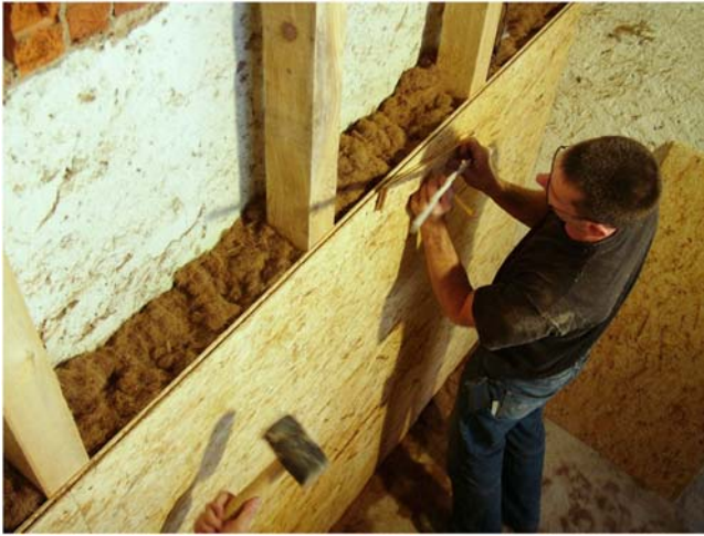
FIGURE 7.3 Algae-based insulation. Courtesy of Neptutherm GmbH.
