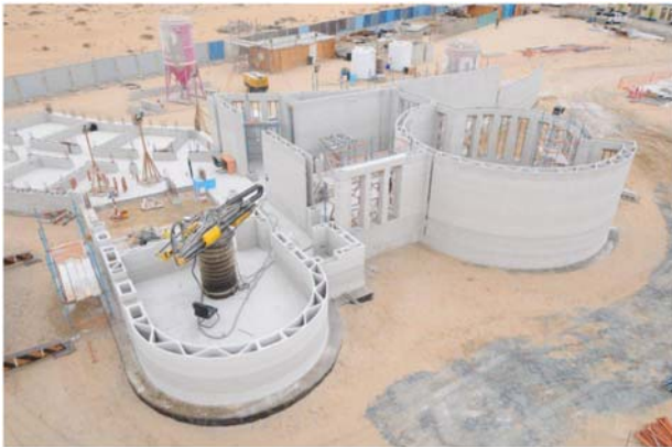
FIGURE 8.39 Building in Dubai 3D printed with Apis Cor. Credit: Apis Cor.
