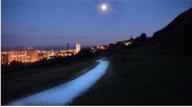
FIGURE 7.36 Photoluminous pavement. Courtesy of Pro-Teq Surfacing Ltd.
