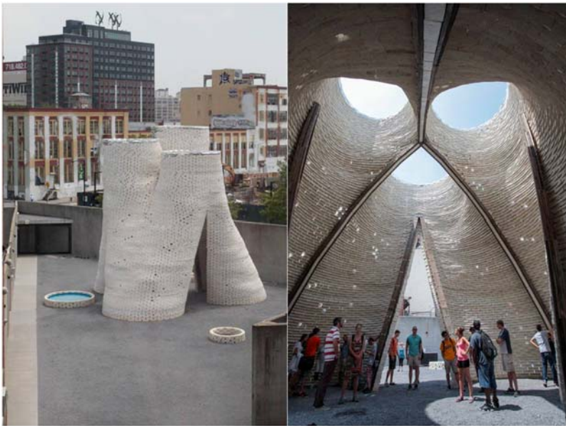
FIGURE 7.6 Hy-Fi, The Living, New York. Courtesy of Ecovative.
