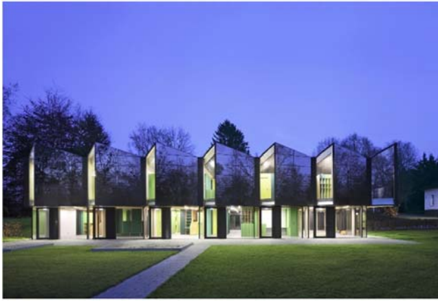
FIGURE 12.9 Nursery + e In Marburg. Courtesy of Opus Architekten.
