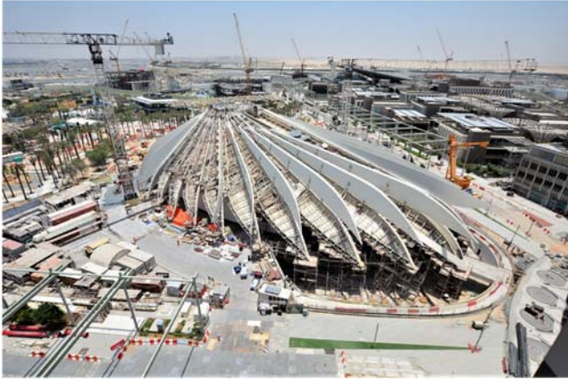
FIGURE 9.15 Drone supervision of UAE Pavilion at EXPO 2020. Courtesy of Santiago Calatrava llc.
