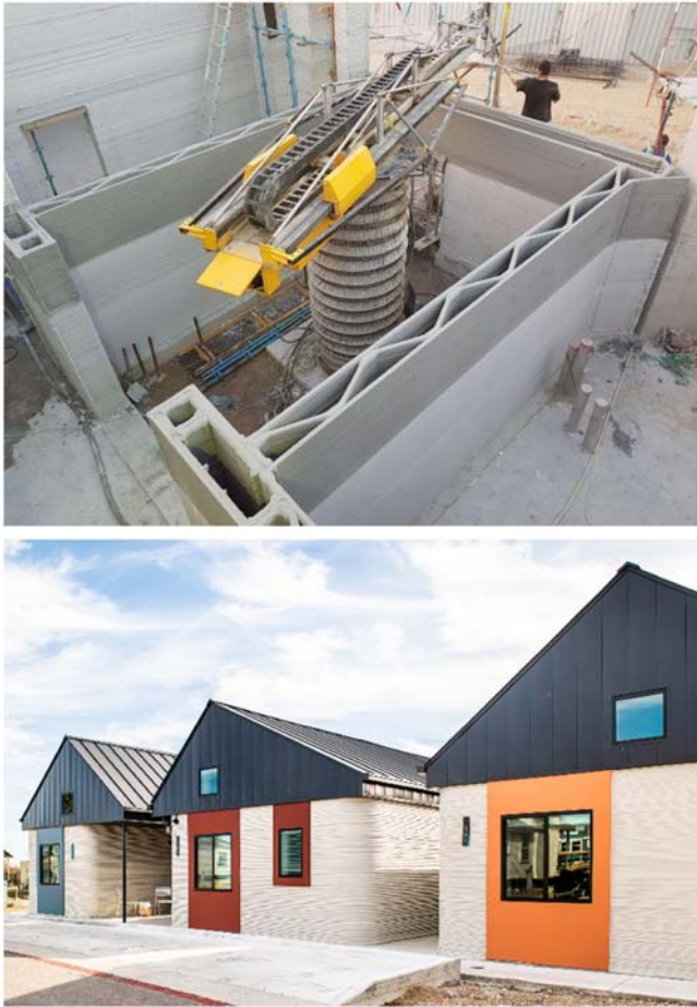
FIGURE 3.12 Buildings scale 3D printing. Courtesy of Apis Cor (top) and ICON (bottom).
