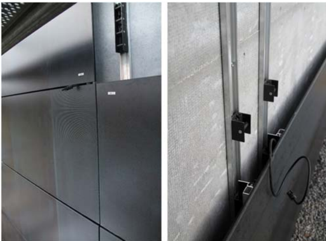
FIGURE 12.13 PV Façade modules installation. Courtesy of Heliartec.
