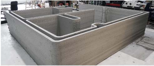
FIGURE 7.10 3D printed concrete walls. Courtesy of COBOD.
