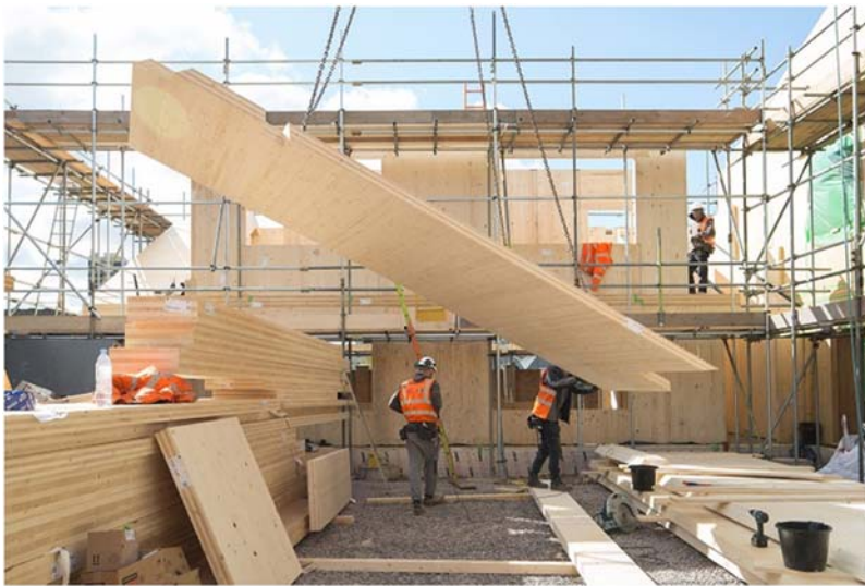
FIGURE 7.13 Assembly of a CLT building structure. Courtesy of Edward Williams Architects, Canducci Group, Agnese Sanvito photographer.
