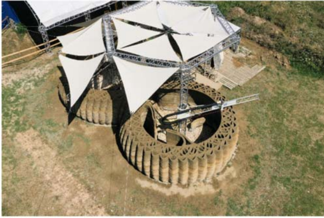
FIGURE 8.38 Crane WASP modular 3D printer building TECLA house. Courtesy of WASP.
