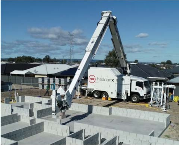
FIGURE 8.8 Hadrian X bricklaying robot. © 2021 FBR Limited.
