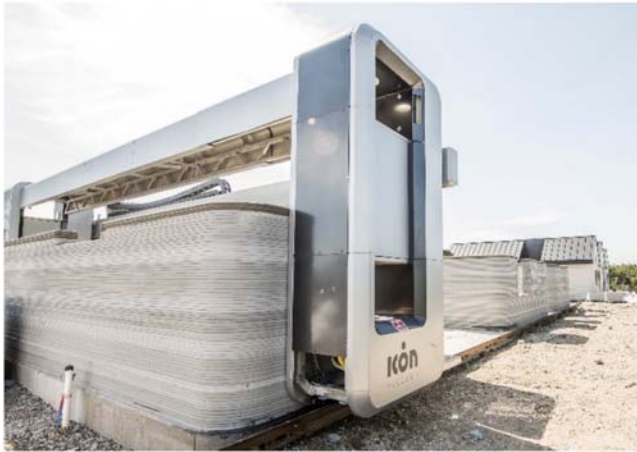
FIGURE 8.40 Vulcan II 3D printer. Courtesy of ICON.
