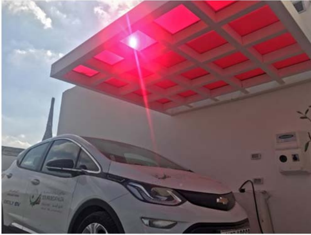
FIGURE 7.52 Canopy with LSC panels of Sapienza University solar house. Photo by the author.
