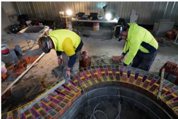
FIGURE 9.27 MR overlay of brickwork guidelines with Hololens. Credit: G. Janh, Fologram.
