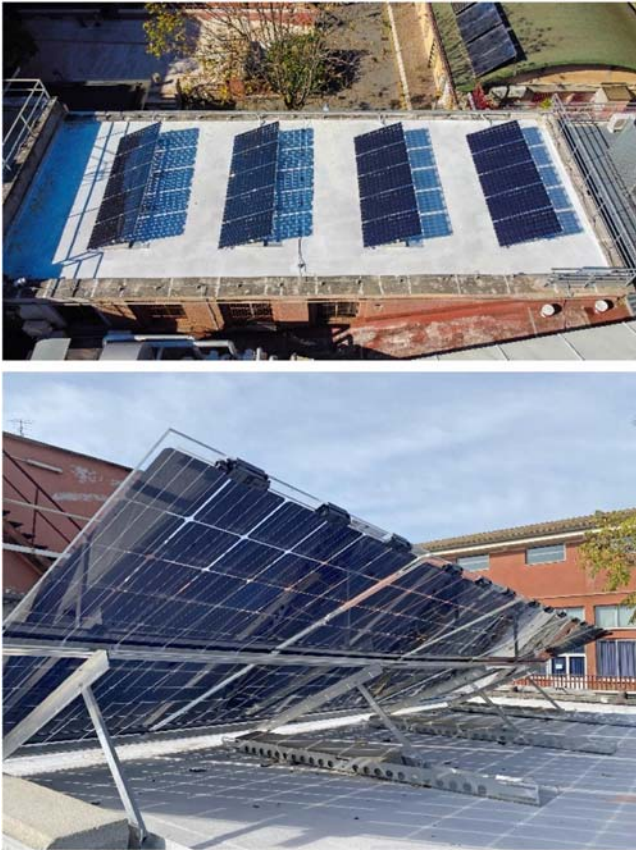
FIGURE 12.18 Bifacial crystalline PV cells. Faculty of Architecture—Sapienza University of Rome. Photo by the author.
