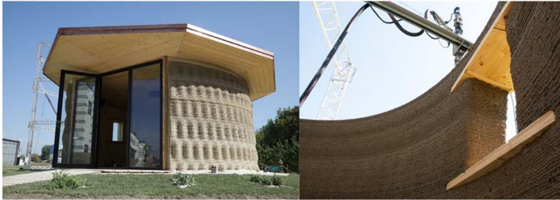
FIGURE 7.11 GAIA 3D printed house with soil, limestone, and agricultural waste. Courtesy of WASP.
