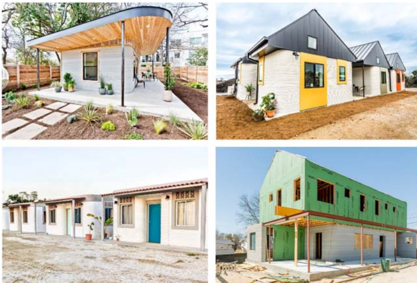
FIGURE 8.41 3D-printed buildings by ICON: first permitted house (top left), community housing in Austin (top right) and Mexico (bottom left), mixed tech house in Austin (bottom right). Courtesy of ICON.
