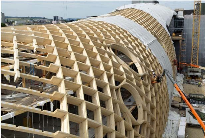
FIGURE 6.52 Construction of Swatch HQ, Biel. Courtesy of Shigeru Ban Architects, photo by Philip Zinniker.
