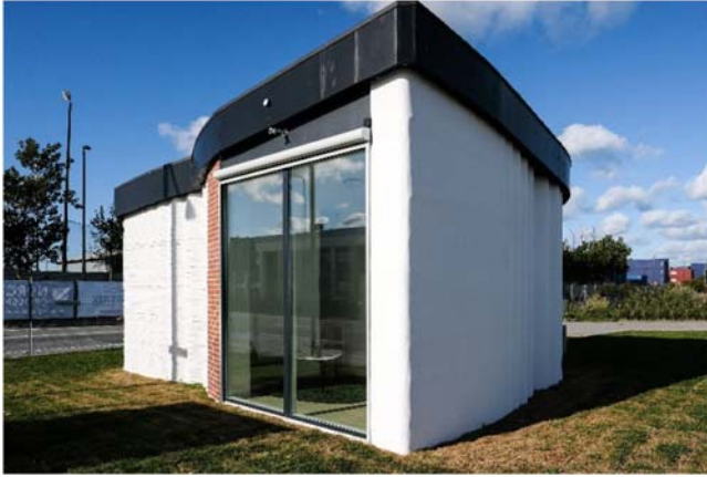
FIGURE 8.42 Building On Demand (BOD) 3D-printed house. Courtesy of COBOD.
