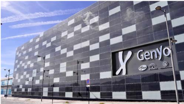
FIGURE 12.16 Semitransparent a-Si BIPV facade, GenYo Centre, Granada. Courtesy of Onyx Solar llc©.
