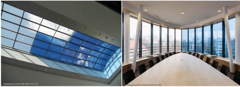
FIGURE 7.24 Electrochromic windows. Courtesy of EControl-glas.
