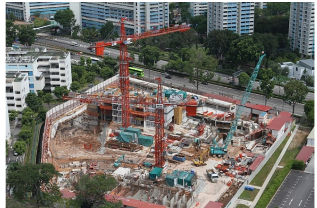
Fig. 6. Tower crane for module lifting [16].
