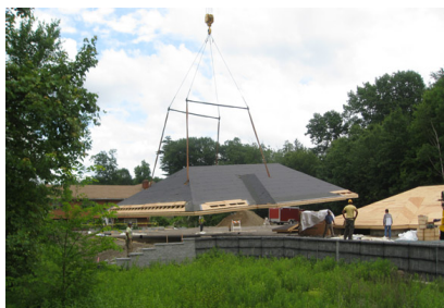
(b) Installation prefabricated Roofs
