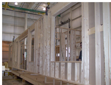
(c) Prefabricated Wall Panels
