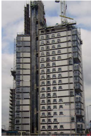
Figure 6: 25 storey student residence in Wolverhampton during construction (courtesy Vision Modular Systems)
