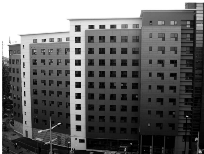
Fig. 6. 12-story modular student residence at Bond Street, Bristol (image by R. M. Lawson)
