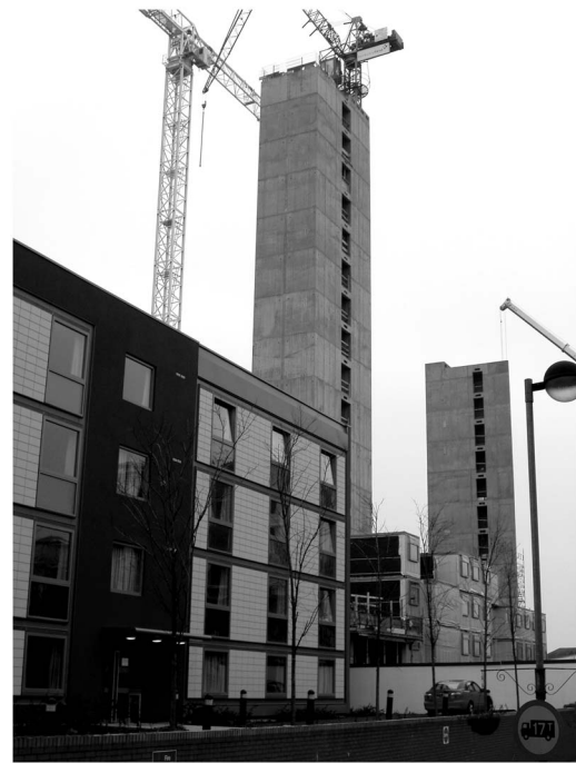
Fig. 4. 17-story modular building stabilized by a concrete core (image by R. M. Lawson)
