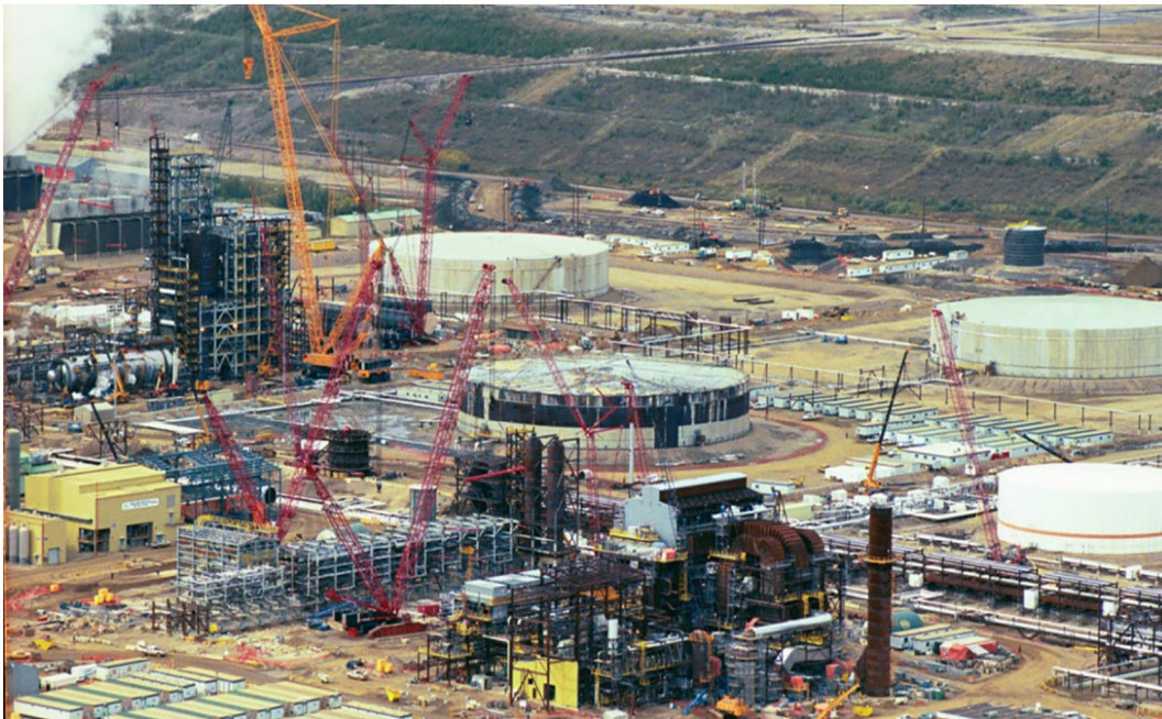
Fig. 1. Modular construction of an industrial plant.
