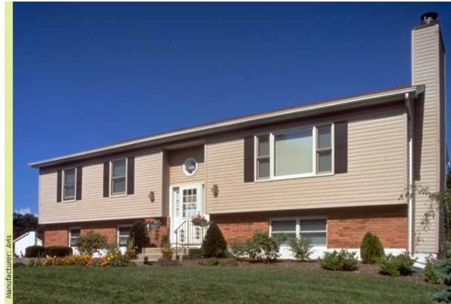
The recessed entry, cantilevered front, and brick kneewall make this a classic American raised ranch
