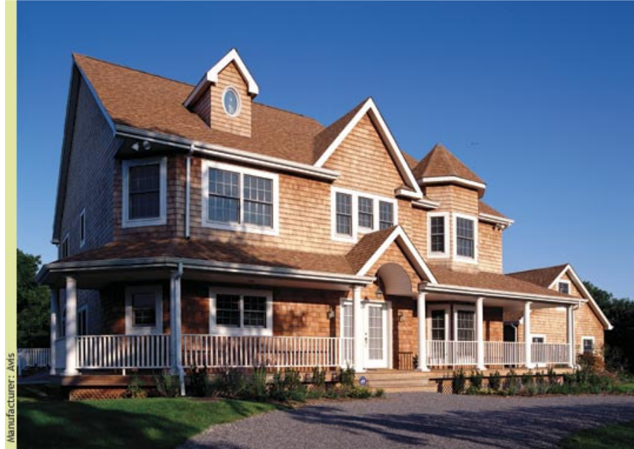
The Victorian features are crafted within the modules, saving on-site work
